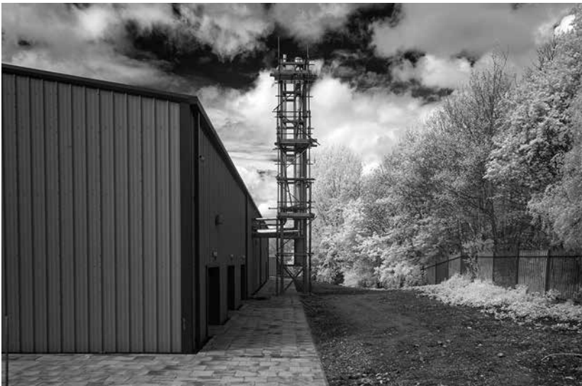
Pipework connecting the River Tyne and heat pump, infrared photograph, Paul Dolan, 2023
