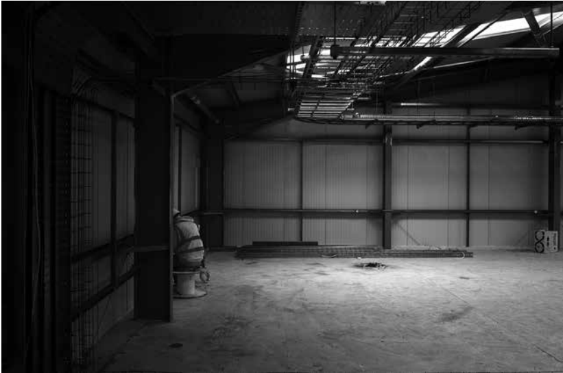
Construction worker in the upper section of the heat pump building, infrared photograph, Paul Dolan, 2023
