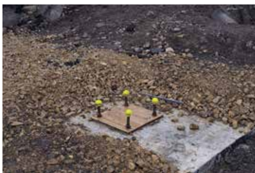
Concrete base built on top of the mine, Hebburn, Paul Dolan, 2023
