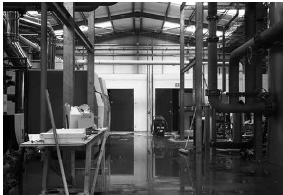
Viking Energy Network water pump building under construction, infrared photograph, Paul Dolan, 2023
