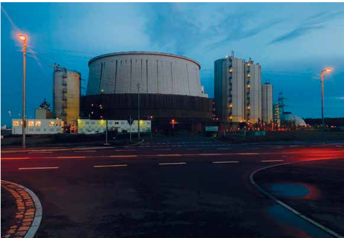
Moorburg Power Plant, Hamburg. Photograph courtesy of Anders Ehlin, The New Liquidity
